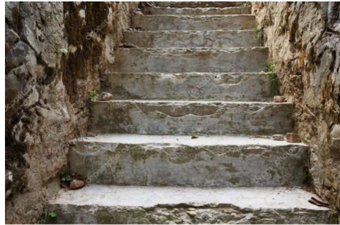
(ii) Stone stair
