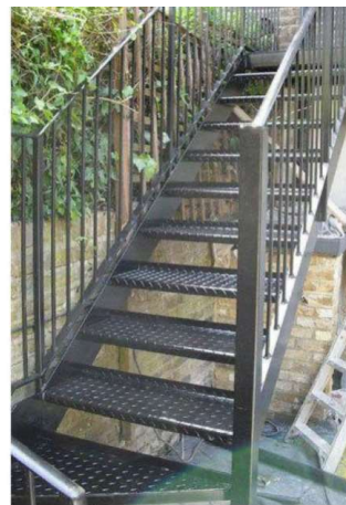
(iv) Metal stair
