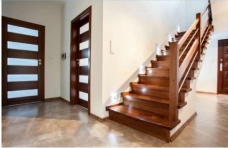
(i) Timber stair
